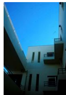
A Void brings both light and air into the rooms on the north side of the building. (Setagaya ward, Fukazawa Symbiotic Housing Project)
